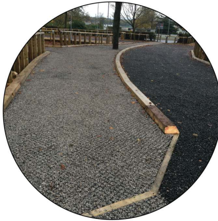
Backfilled with gravel
